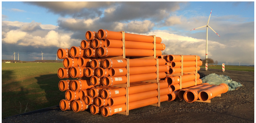
Fig. 15 – 375mm and 400mm orange sewage pipes waiting to be installed
