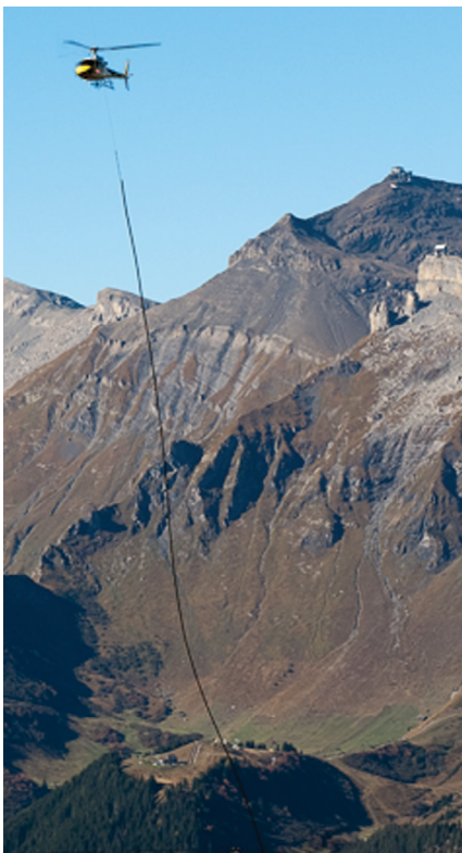
Fig. 4 – Pipe transport by helicopter
