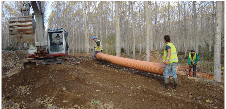
Fig. 14 – Corrugated pipes made from Hostalen PP H2464 – courtesy of PLOMYPLAS
