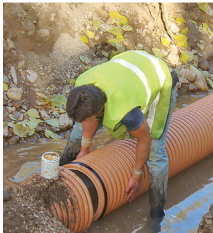
Fig. 16 – Push connection, inline socketing courtesy of PLOMYPLAS
