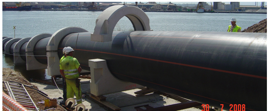
Fig. 5 – Seaoutfall line – courtesy of PLOMYPLAS
